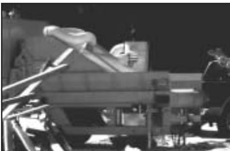
Gypsum wallboard grinding unit equipped with an air filtration device to control dust emissions during grinding activities. The large pieces of gypsum wall board are being loaded onto the belt for processing.
