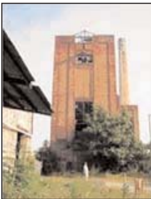
AMBLER BOILER HOUSE BEFORE
