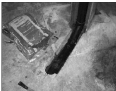
Suction cavity with HDPE piping
