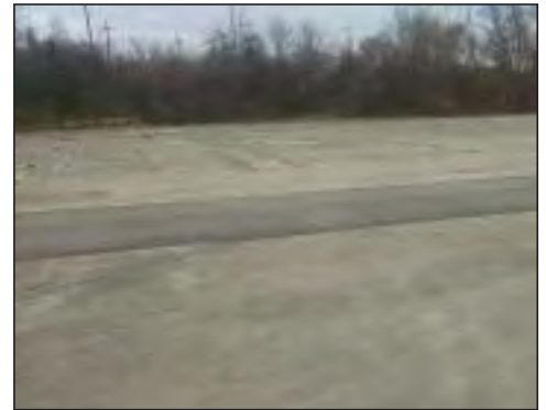
Former Building Acting as a Cap
